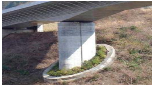
Figure 5 Photo of bamboo-cutting method of shaft foundation
