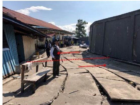
Figure 7 Offset Rupture 4,8 m at desa Donggala Kodi, Ulujadi, Palu city, Central Sulawesi
