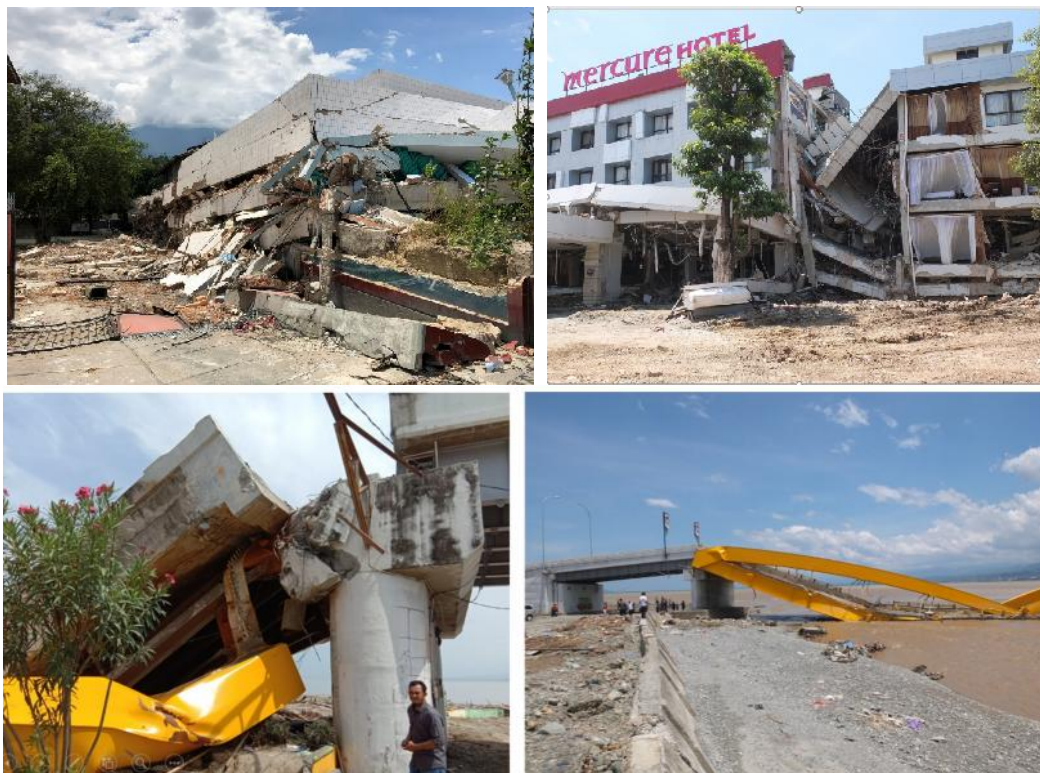
Figure 10 Building and bridge damages induced by earthquake in Palu
