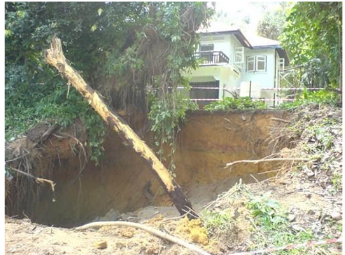
Figure 10 Sinkhole over a slurry TBM working in a mixed face of soil and rock grades of weathered Singapore granite
