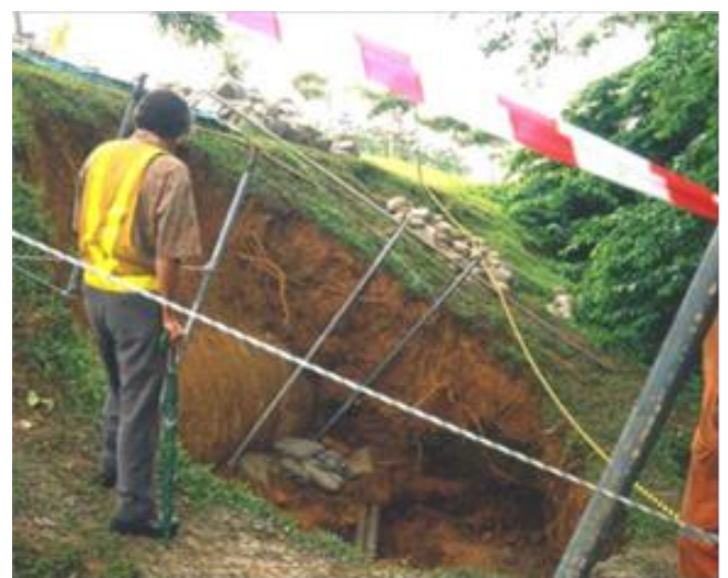
Figure 7 Sinkhole over an EPB working in mixed soil and rock grades of weathered Singapore granite
