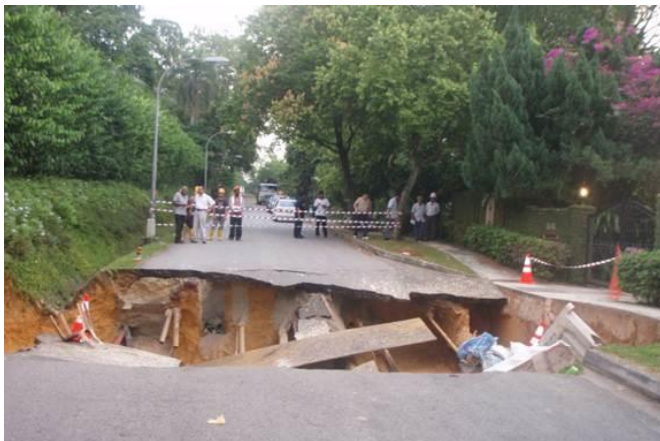
Figure 9 Sinkhole over a slurry TBM working in a mixed face of soil and rock grades of weathered Singapore granite
