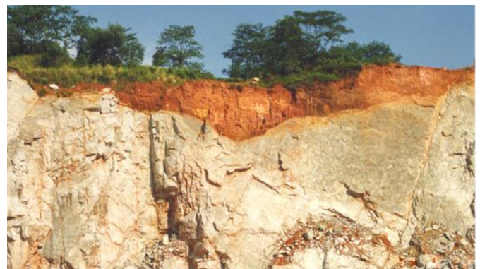
Figure 1 A rock head profile in weathered Singapore granite
