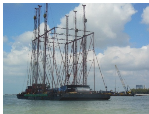
Offshore PVD Installation
