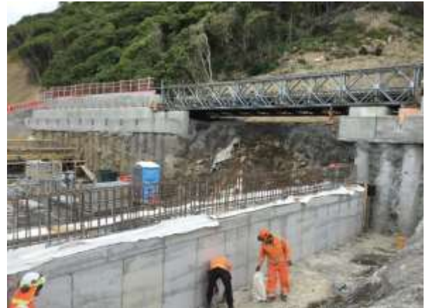
Figure 9- Bailey bridge installed above the bored pile retaining wall to enable traffic to pass safely, during the RTW 3 and debris flow bridge construction
