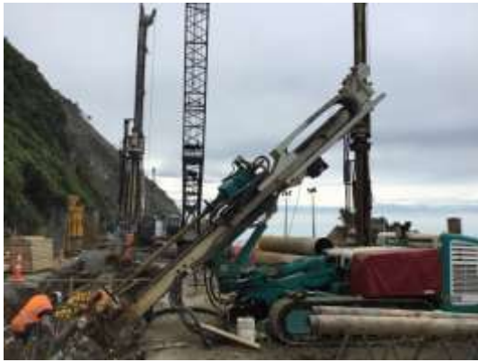
Figure 10-Bored pile construction (at RTW 3D1, an anchored section of RTW 3
