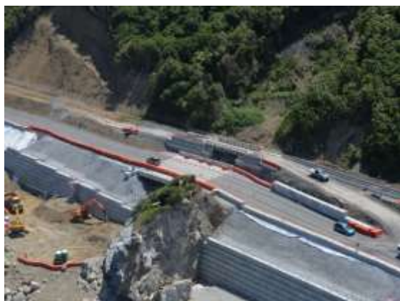
Figure 11-State Highway 1 opened after road debris flow bridge construction, the debris flow channel construction underway.
