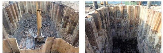
Figure 15 Excavation inside the cofferdam
