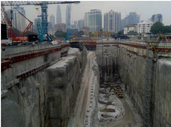
Figure 6 Excavation works at TRX station
