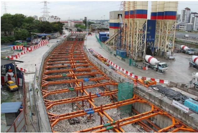
Figure 12 Maluri Portal with strutting support
