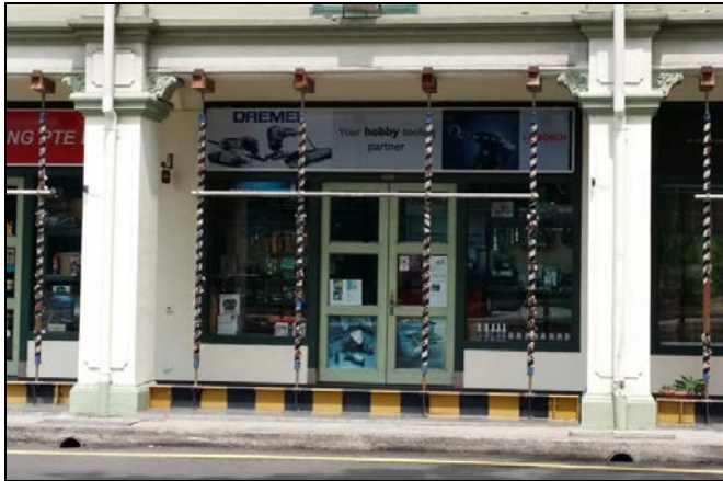
Figure 10 Typical arrangement for building protection propping
