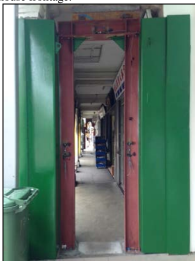
Figure 12 Five-foot way protection system
