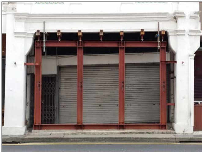
Figure 11 Typical enhanced external building protection measures
