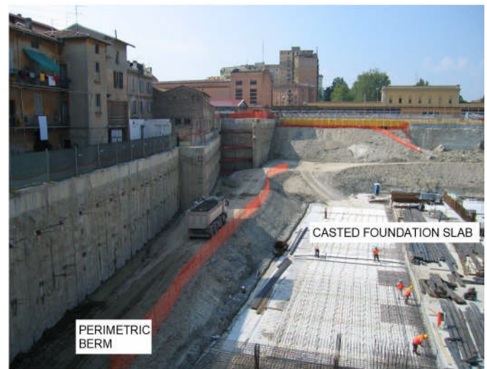
Figure 13A Excavation and execution of r.c. foundation slab
