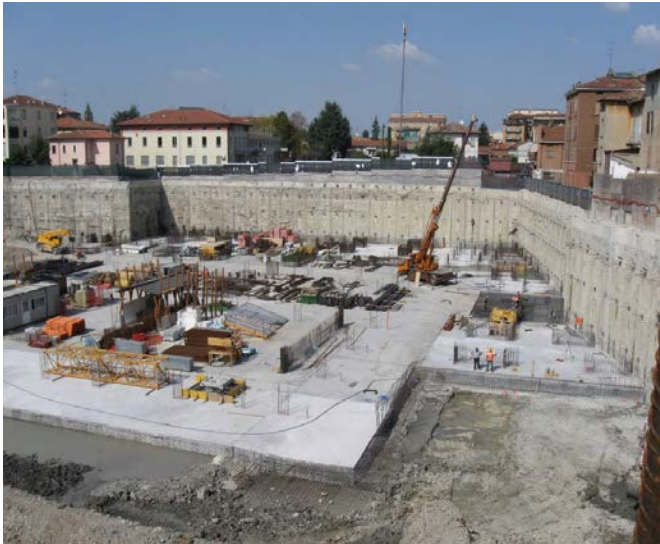
Figure 13c Last excavation phase in east side diaphragm wall
