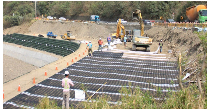
Figure 5 The Installation of GRS
