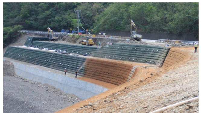
Figure 7 Hydroseeding
