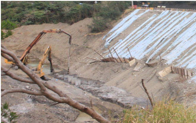
Figure 3 The All-Casing Pile Installation
