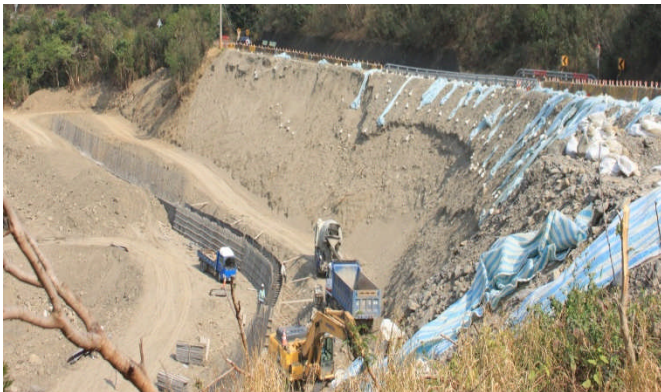
Figure 4 Semigravity RC Retaining Wall Construction
