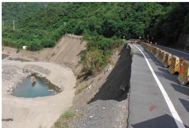
Figure 1 Slope Failure below Highway Embankment
