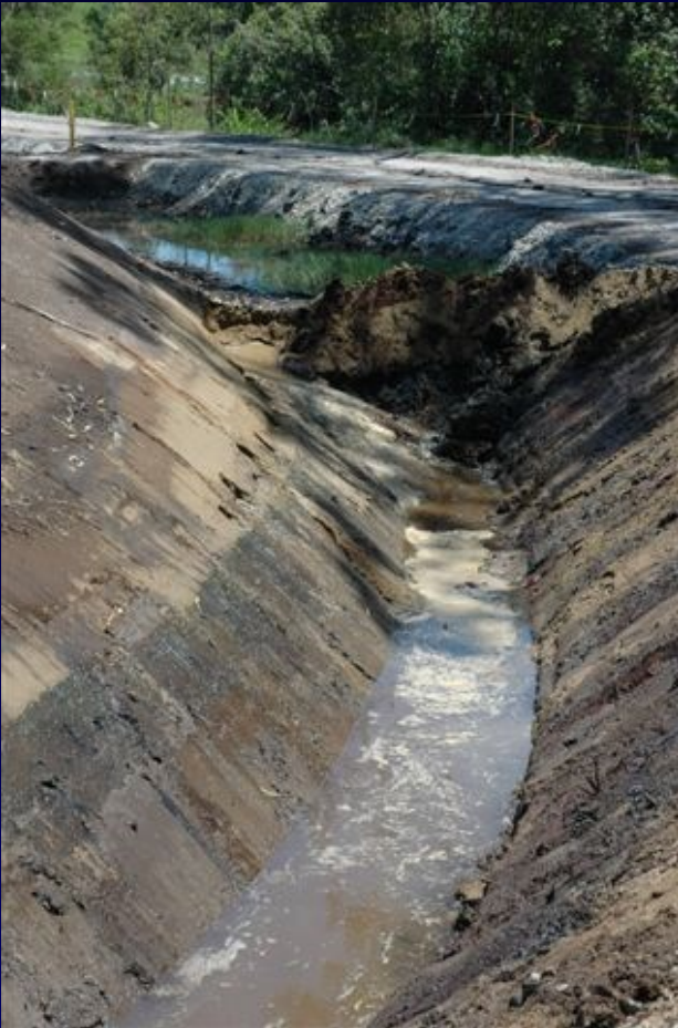
Peripheral bentonite trench
