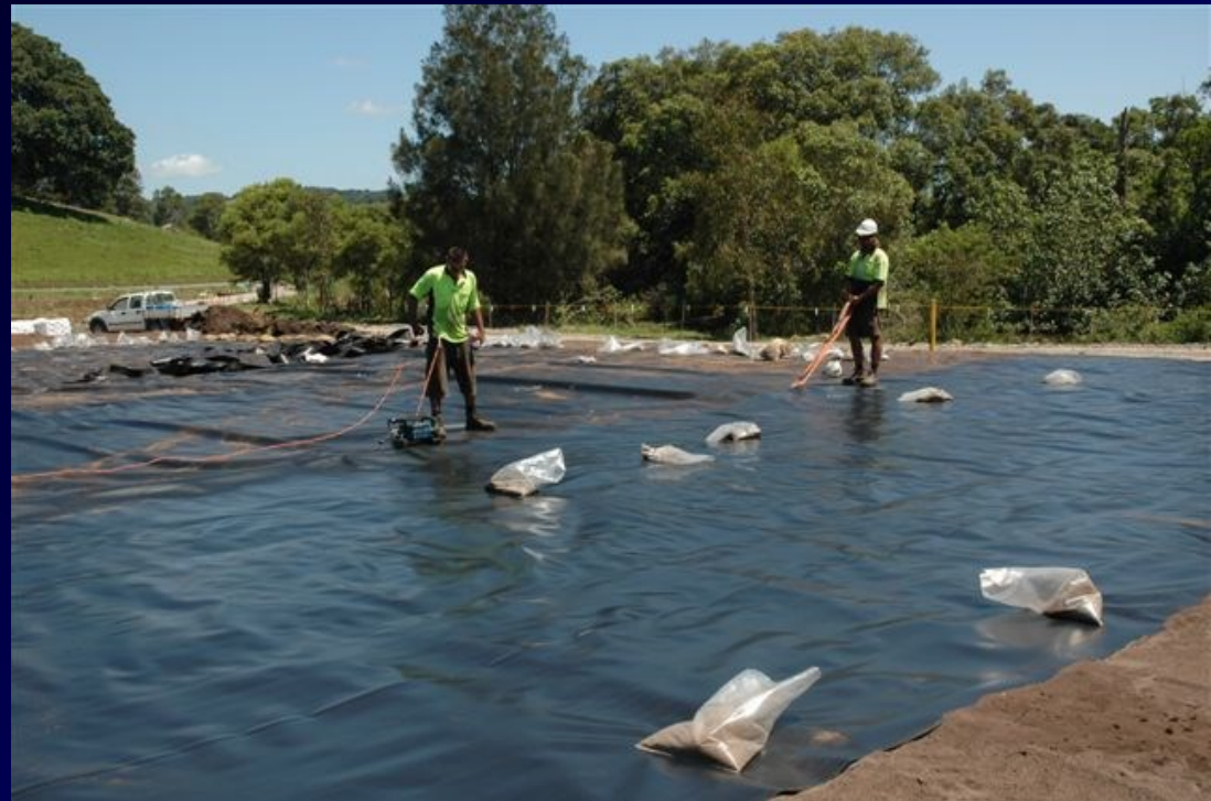
Membrane installation
