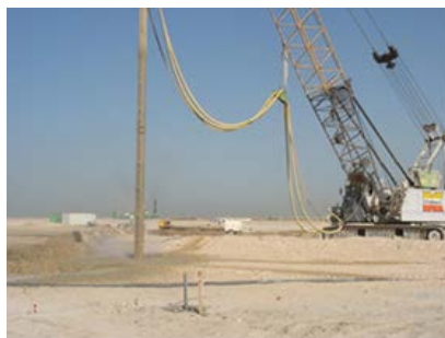
Fig. 5: Deep Vibrocompaction at 3.85m Triangular Grid Centres
