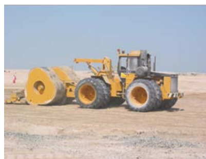
Fig. 6: Landpac Compacting Near Surface layers
