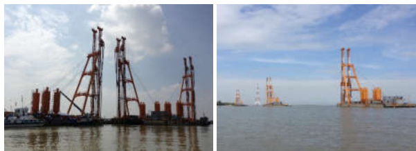
Photo 3 CDM Installation Work
