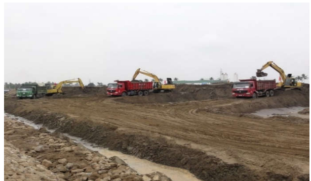
Photo 9 Surcharge Filling Work
