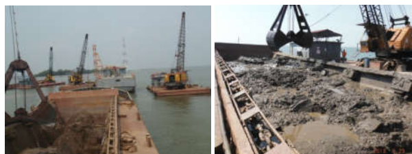
Photo 4 Dredging work until CDL -2.0 m
