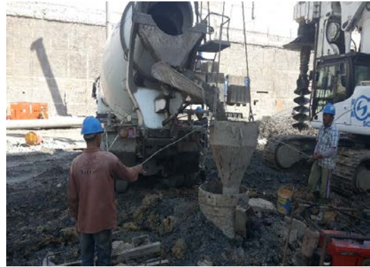
Figure 20 : Concreting of boredpile with tremie
