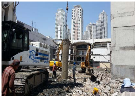
Figure 18 : Use of casing for bored pile
