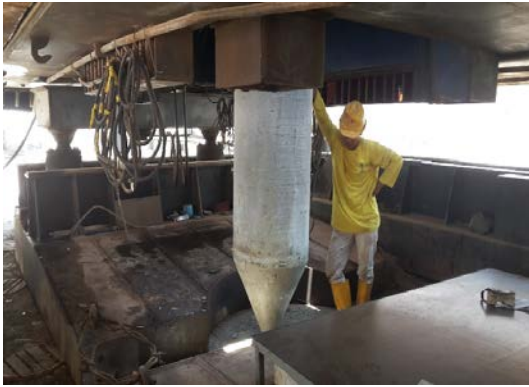
Figure 16 : Preparation for Pile Injection
