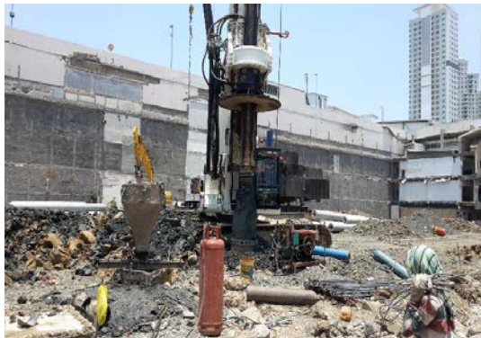
Figure 17 : Installation of Boredpile
