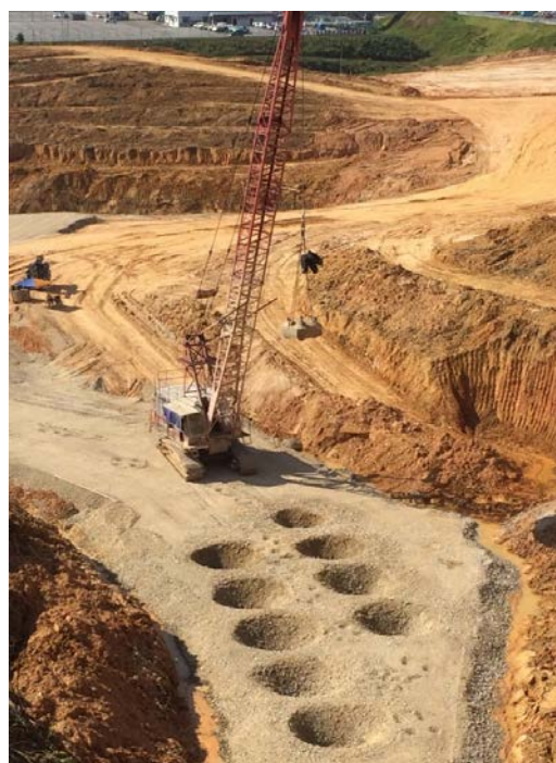
Figure 3 DC rig setup for deep valley compaction
