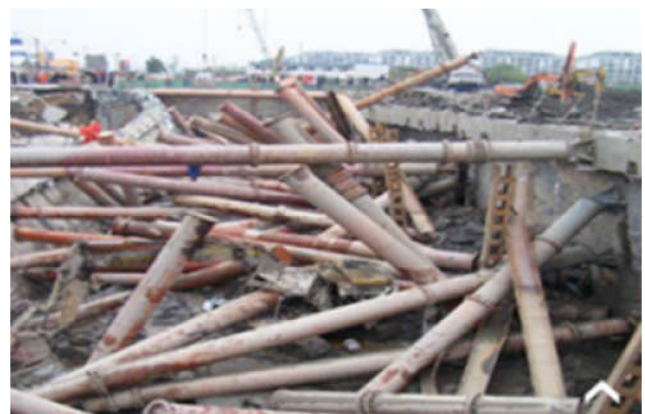
Figure 2 Failure of excavation
