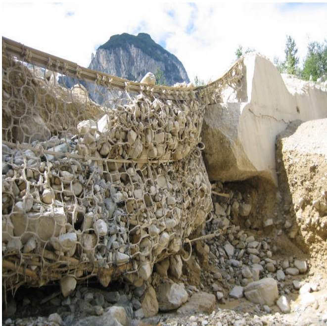
Figure 11 Washed out anchoring of the debris flow barrier number 25 in the Illgraben channel. Anchoring partially in loose material and partially in disused concrete debris flow barrier
