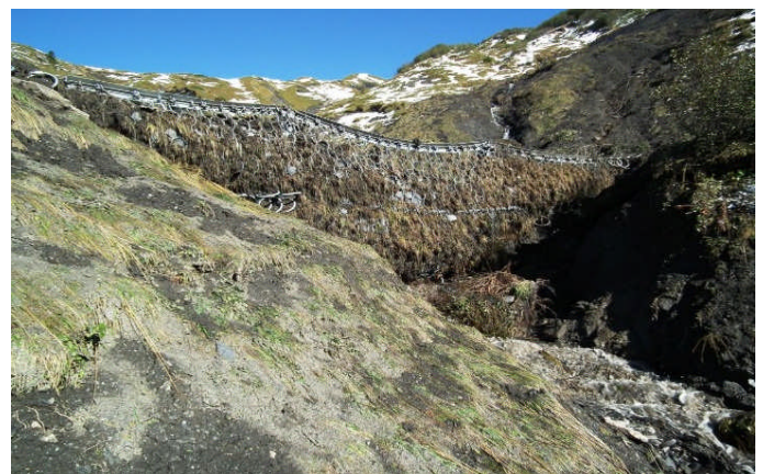
Figure 16 11 debris flow protection barriers, successfully filled in Hasliberg in 2011
