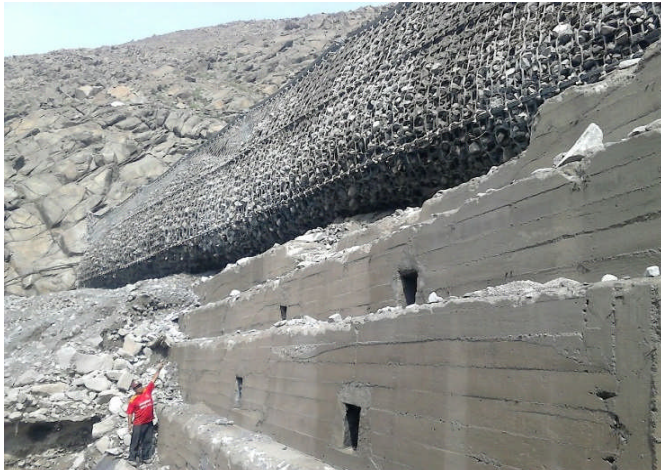
Figure 17 Filled debris flow barrier in 2017 in Chosica Peru, protecting successfully a large city downstream
