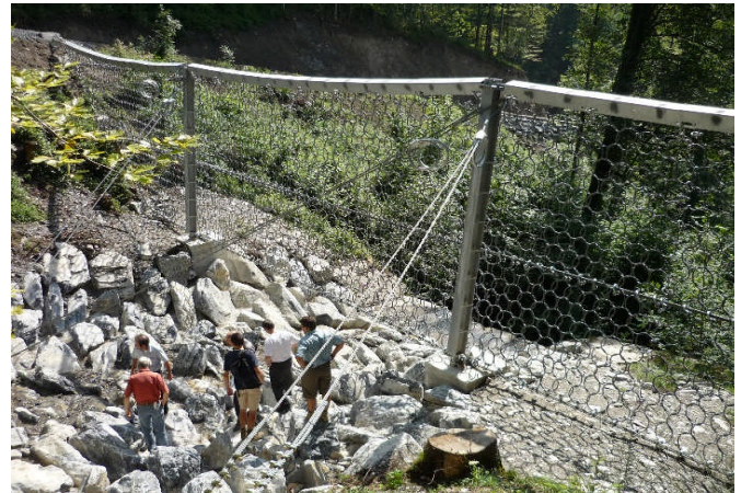
Figure 4 UX debris flow barrier, with posts for wider stream channels application. Example of the Trachtbach in Switzerland. Additional kolk protection, rip-rap and lean concrete were placed along the stream bed
