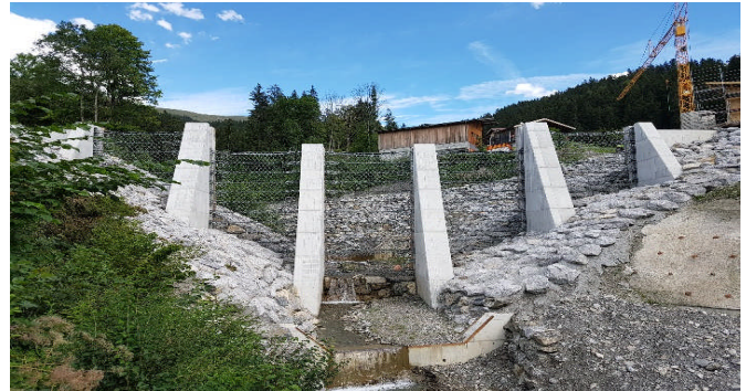
Figure 19 Another special construction acting as a debris flow barrier in Sitäbach consisting of concrete slices piled up and netting mounted in between
