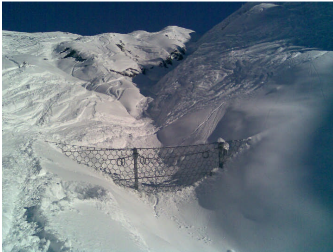
Figure 10 Barrier partially snowed in during winter. The snow load must be considered for designing
