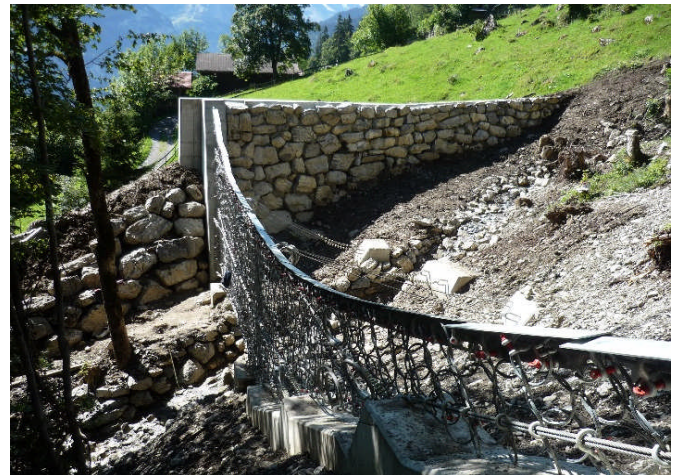
Figure 15 Debris flow barrier in Isenflue above a settlement. The outer bank of the stream was reinforced with a rock wall
