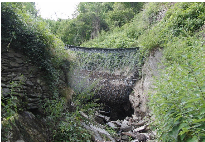
Figure 14 partially filled debris flow barrier above the German Railway close to Koblenz
