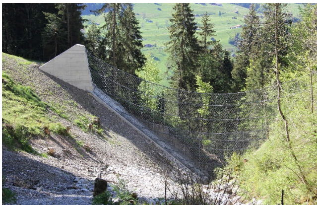
Figure 18 Special construction of a debris flow barrier in Hüpach, in Switzerland, with a width of 40 m and a netting height of 10 m
