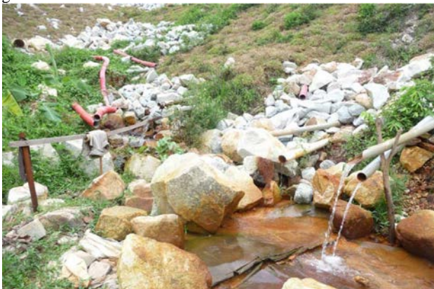
Figure 3 Copious flow of water seeping out from the toe of embankment
