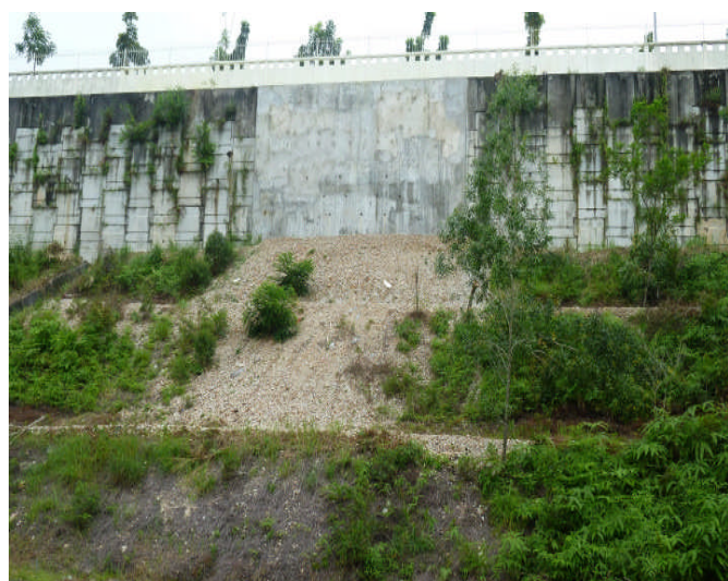
Figure 12 Short term remedial work using RC wall
