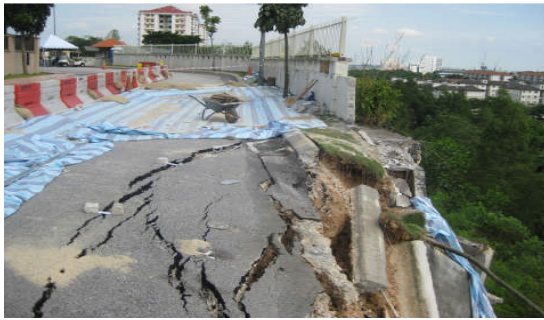
Figure 2 Partial collapsed of reinforced soil wall on 20 th May 2011
