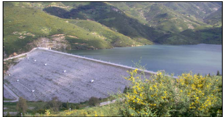
Figure 1a General view of El-Agrem concrete face rockfill dam
