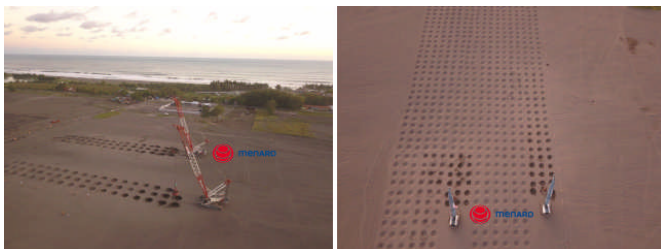
Figure 15 Dynamic compaction work on site
