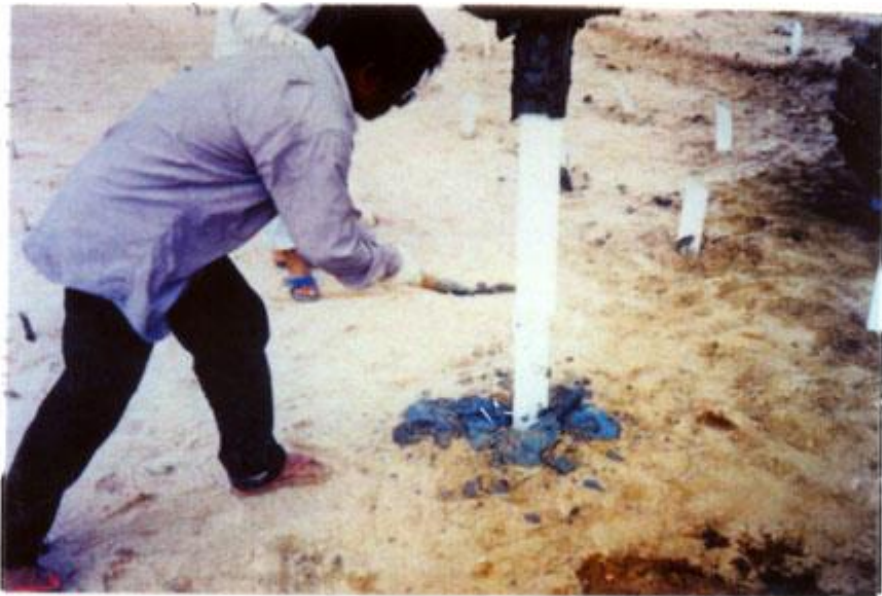
Fig. A-20 PVD Installation in Field
