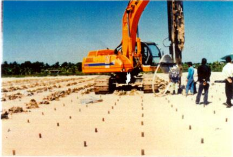
Fig. A-19 PVD Installation in Field
