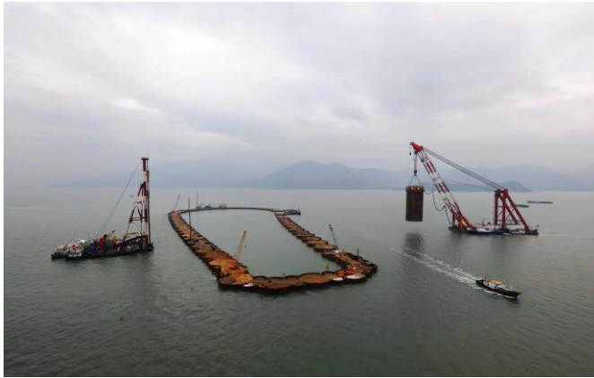
Figure 11 East artificial island cofferdam construction
