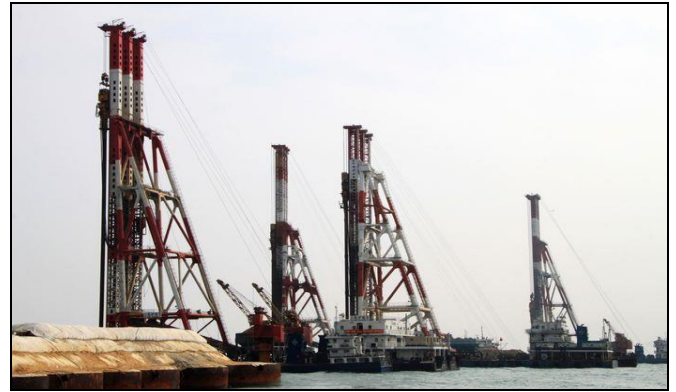
Figure 19 Sand compaction pile (SCP) application
