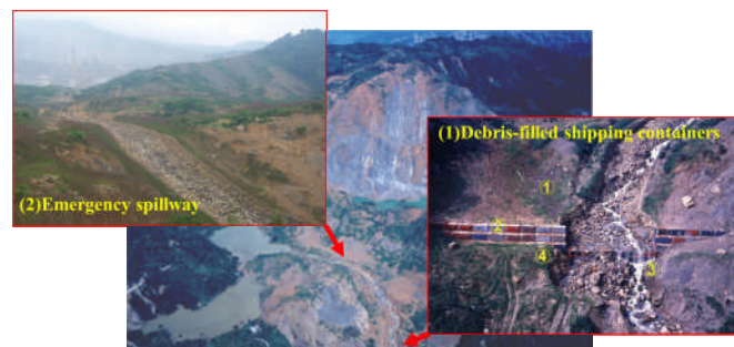
Figure 5 Locations and photos of emergency treatments in the landslide
