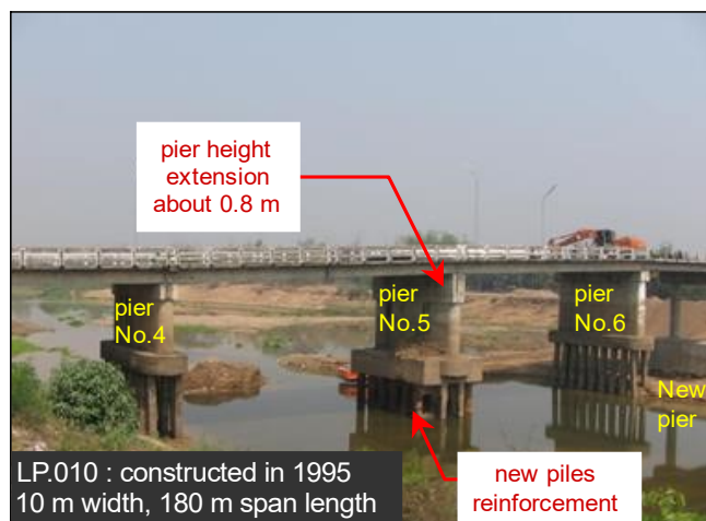
Figure 3 Repair of the settled bridge LP.010 in Lamphun, Thailand (2008)
