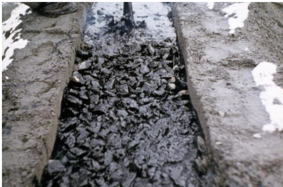
Fig. 2. Injecting hot bitumen into gravel matrix
