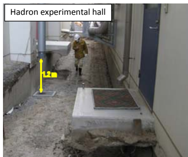
(a) Ground subsidence along building
