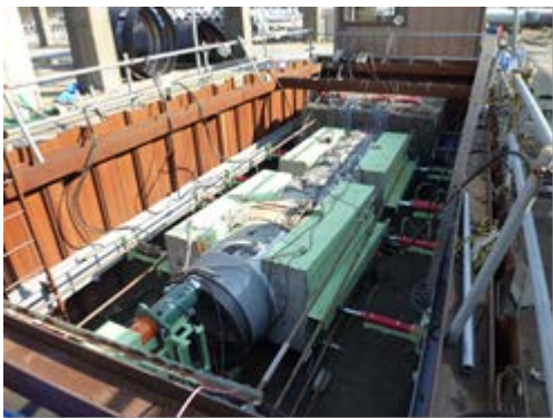
Pipe Jacking (after Le et. al, 2013)
