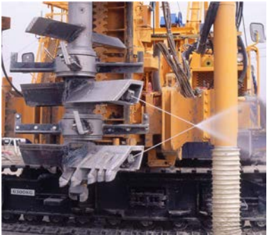
3. Deep mixing using High Pressure Jet Grout (after Kitazume, 2013)
