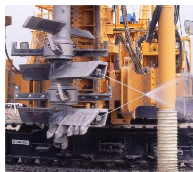
3. Deep mixing using High Pressure Jet Grout (after Kitazume, 2013)
