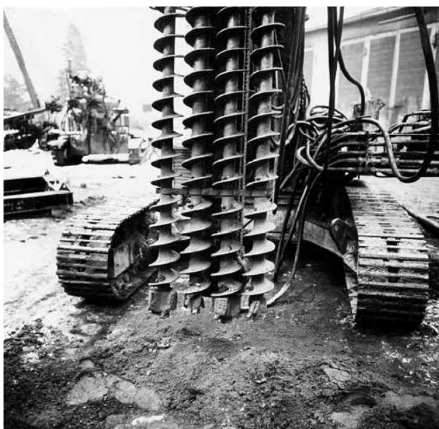
Fig. 7. The first application of Mixed-in-place (MIP) piles, (Stocker and Seidel, 2005).
