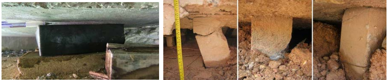
Case 3: Bridge Abutment Distresses due to Piled Embankment Failure
