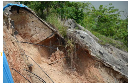
Case 4: Unreliable Facing Capacity of Shrinking Soil Nail Strengthened Slope
