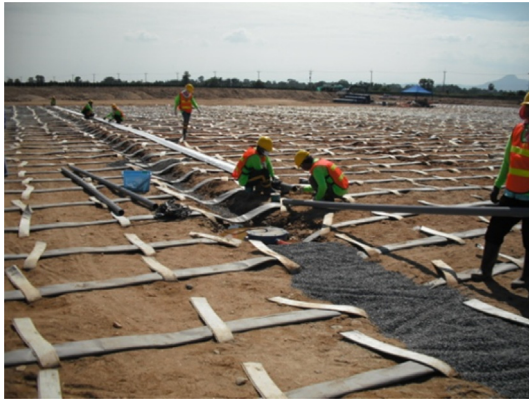
Fig. 8. Installation of horizontal band drains and perforated pipes.
