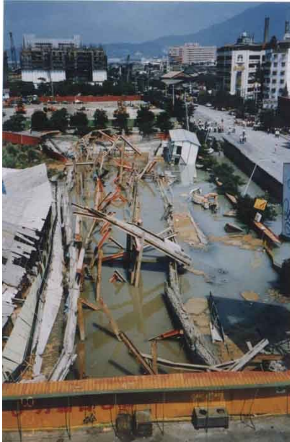
力霸百老匯 excavation failure
