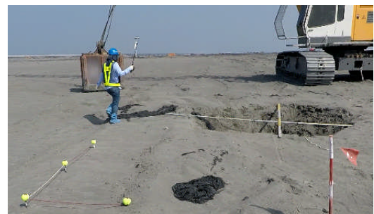
Figure 15. Images acquisition process after-pounding
