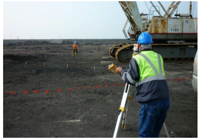
Figure 5. Field surveying work for ground heave and crater volume
