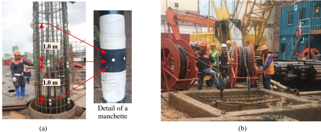
Figure 3 Performance of shaft grouting by FCS: (a) steel cage with grouting tubes; (b) grouting in progress
