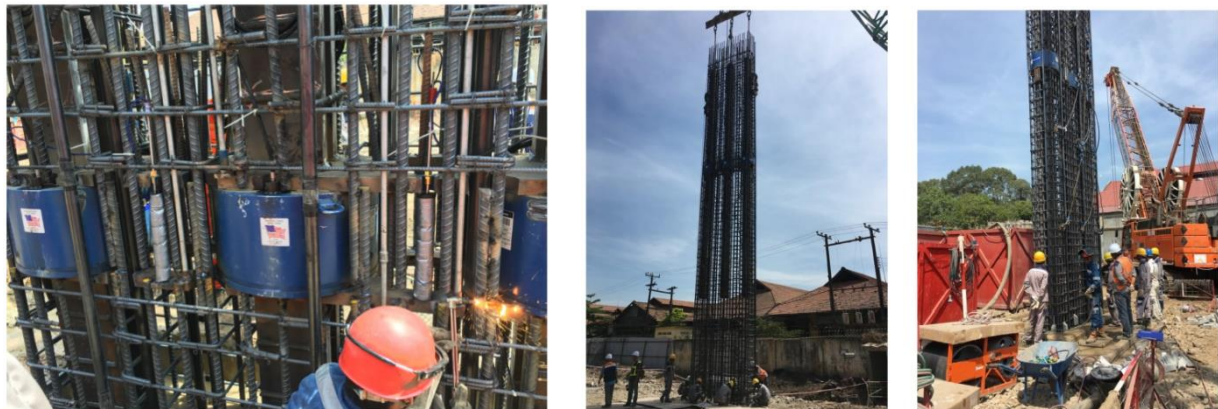
Figure 6 Installation of the instrumented barrette (TN6) at Vinhomes - Bason project
