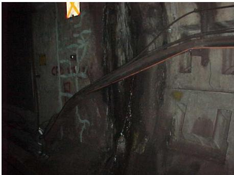
Figure 18 Leakages from tunnel segments with butyl rubber sealing strips after more than 10 years of its construction
