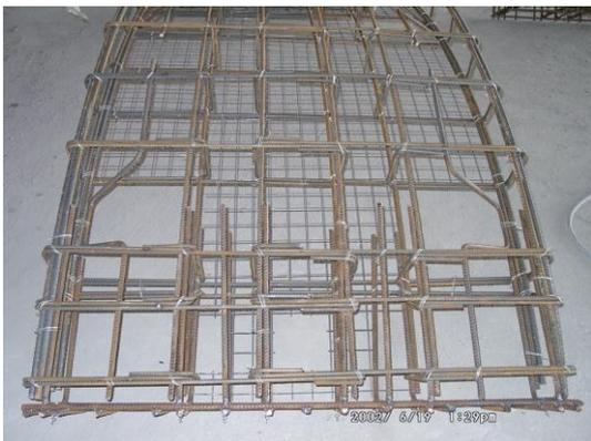
Figure 14 Steel cages with links spaced at 300mm and a wire mesh at the intrados of the segment
