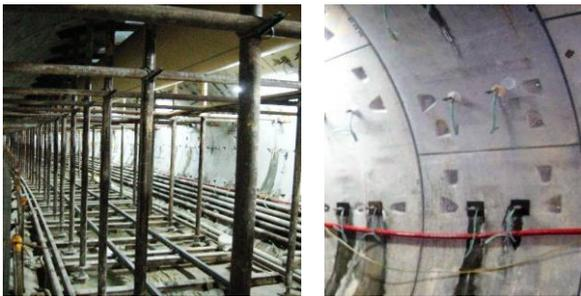
Figure 11 (b) Installed passive support in the first tunnel and GFRP dowels installed through the segments of the first tunnel (Osborne, et al 2008)
