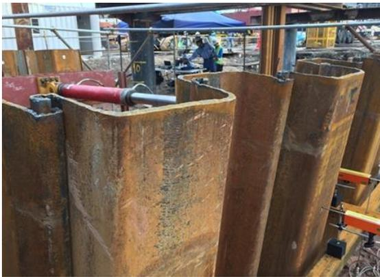
Figure 8 Interlock slippage at the top portion of the IV-pile wall
