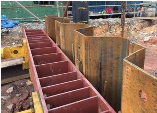
Figure 9 Top portion of the 25H-pile wall
