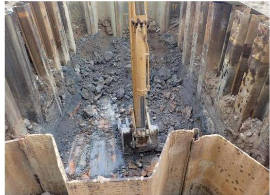
Figure 30 Cofferdam excavation
