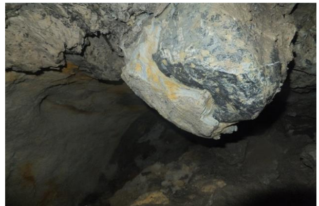
Figure 8 Shield construction face limestone protruding
