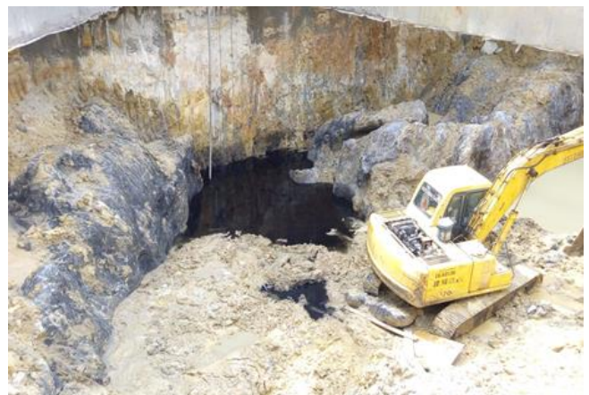
Figure 1 Karst cave encountered during excavation of an underground project in Guangzhou Metro
