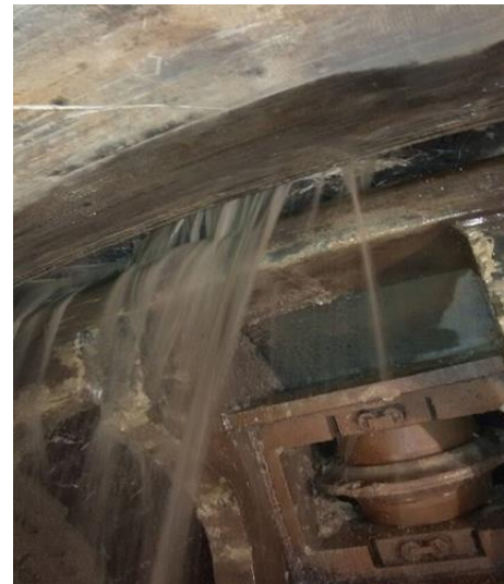
Figure 4 Water gushing from shield excavation face in Karst stratum
