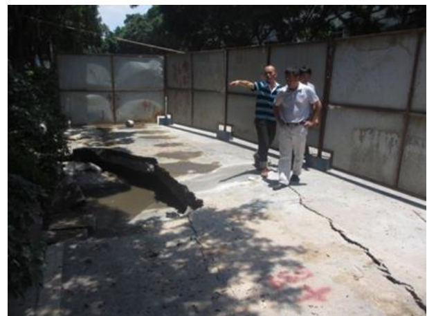
Figure 5 Road subsidence caused by shield construction in Karst Development Area
