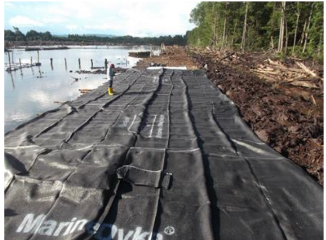
Figure 44 Laying of the geotubes on top of the corduroy.
