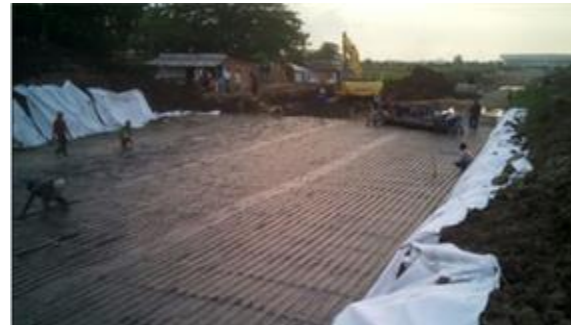
Figure 27 Separator geotextiles and basal geogrids reinforcement.
