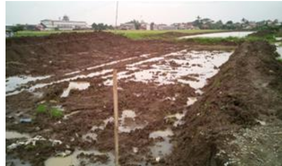
Figure 26 Removal of the 3m soft clay.
