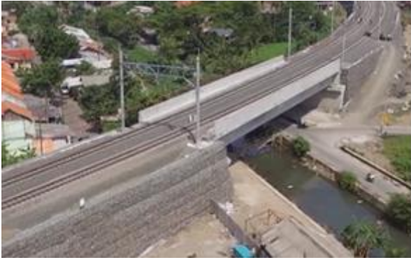
Figure 30 Completed MSE wall construction.
