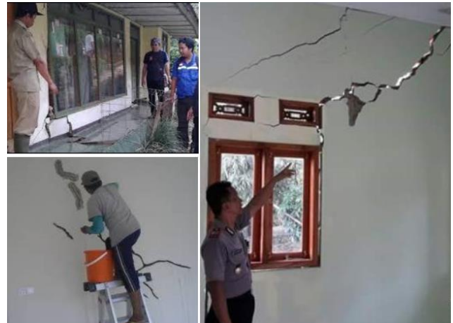
Figure 22 Cracks on houses due to expansive soils.
