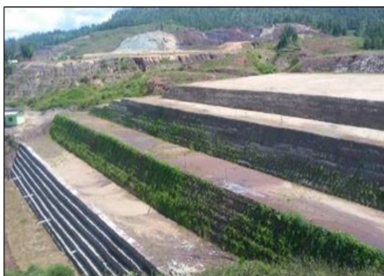
Figure 39 Completed HRSS wall with vegetation on the wall face.
