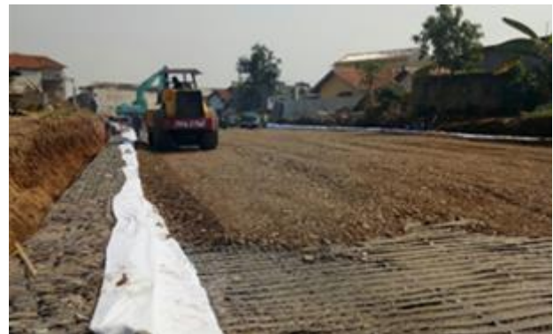
Figure 28 Compaction and building up the embankment.
