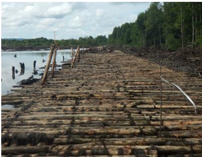
Figure 43 The Corduroy made of three layers of mangrove trunks.
