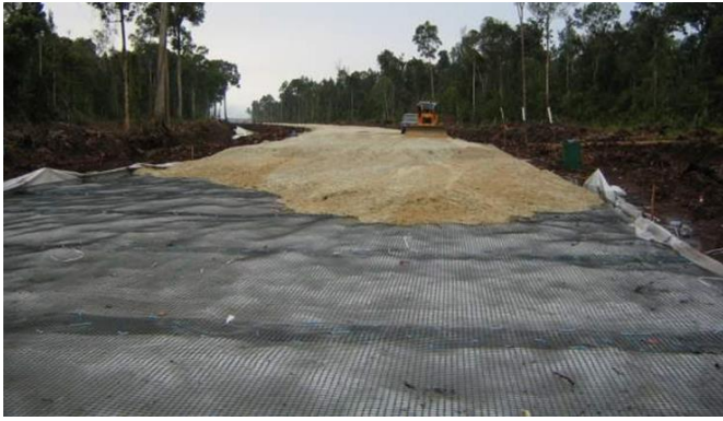
Figure 7 Geosynthetic reinforced road embankment over peat swamps
