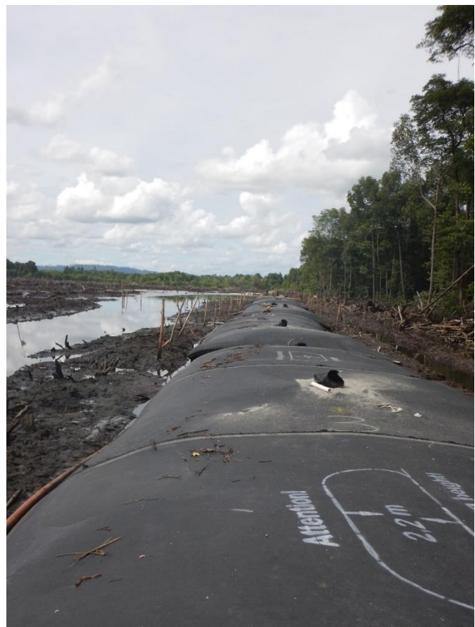
Figure 45 Completed geotube dyke.
