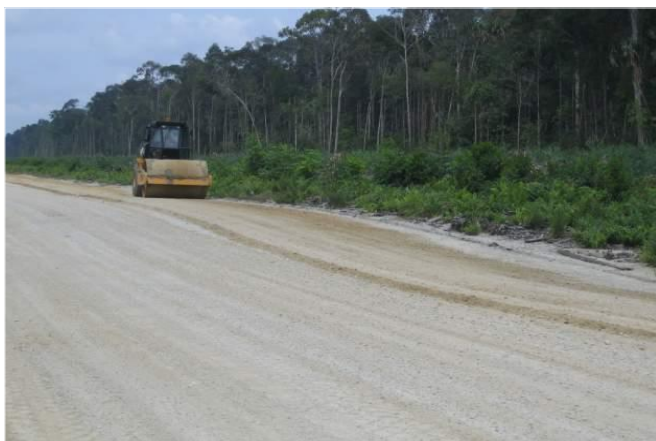
Figure 9 Regrading and re-compaction required from time to time.
