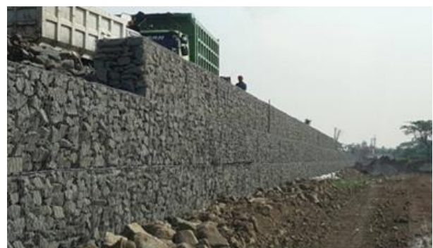
Figure 29 Partly completed anchored gabion facings.
