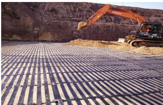
Figure 38 Laying the high strength geogrid and backfilling.
