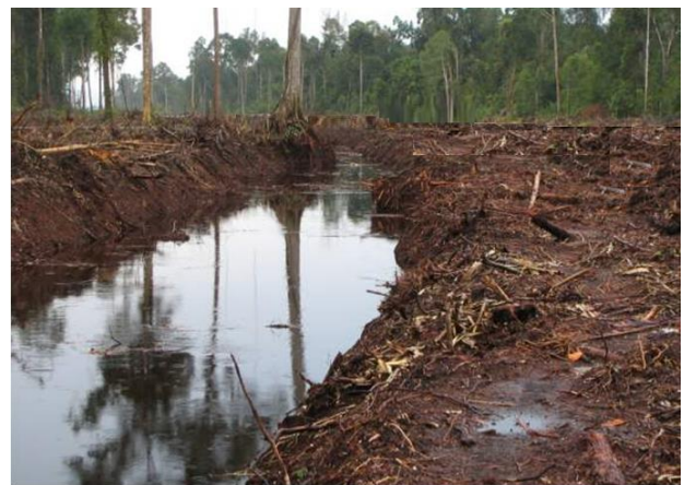
Figure 5 Excavating along both sides of road alignment and forming low peat embankment
