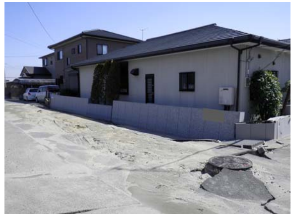
Photo 1 Liquefaction damage of house
