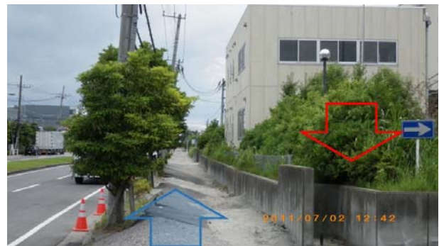
Photo 11 Uplift of public sidewalk as a consequence of liquefaction-induced subsidence of private building
