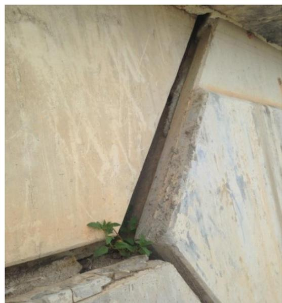
Figure 1 Photo of a dislocated facing panel in Nibong Tebal, Penang
