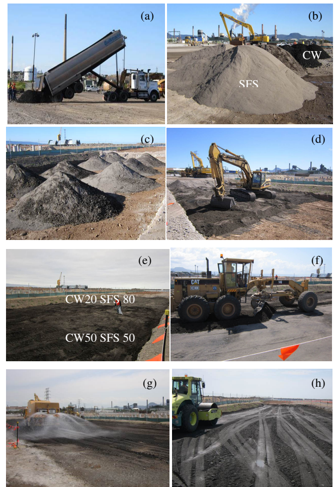
Figure 8 Photos of the field trial (a) arrival of the material on site, (b) stock pile of steel furnace slag and coalwash, (c) mixed materials ready for (d) spreading, (e) sampling prior to compaction, (f) levelling, (g) adding moisture and (h) compaction
