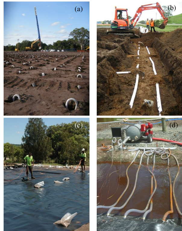
Figure 3 Field trial (a) drain installation, (b) horizontal drain installation, (c) membrane installation and (d) connection between horizontal drainage and vacuum pump (Courtesy of Austress-Menard)
