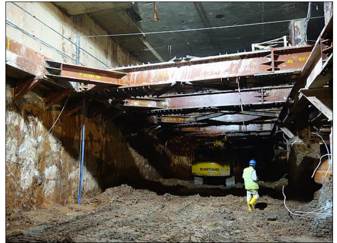
Figure 20 Bukit Bintang Station, Top-up excavation in progress at the lower platform level.
