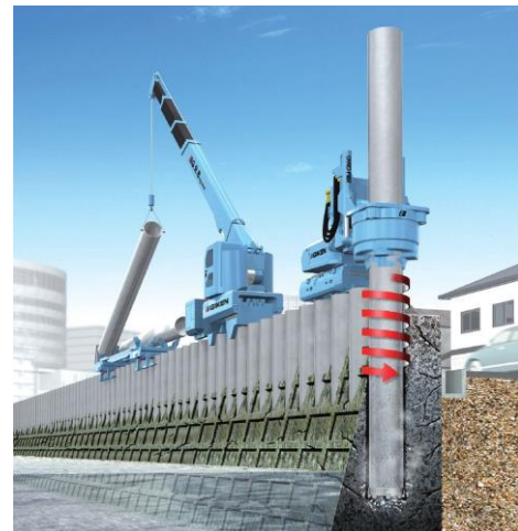
Figure 13 Rotary Cutting Press-in Method
