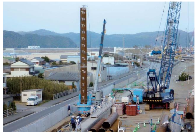
Figure 23 Situation of construction of single pile wall in Nii section
