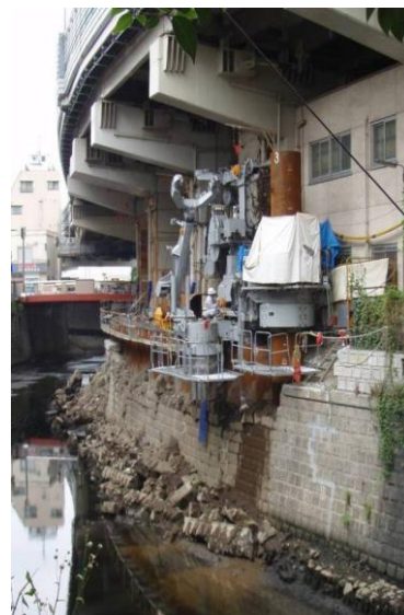
Figure 5 Renovation of revetments under highway bridges
