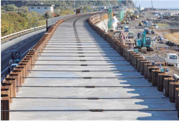
Figure 18 Connection of two walls by tie rods
