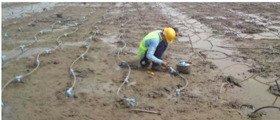
Figure 8b Tubing system of VCM-DT
