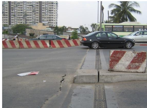
Figure 7 Differential settlement at approach to bridge
