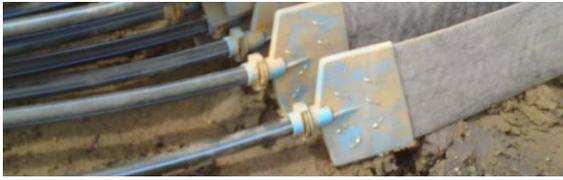
Figure 8a Connection of PVD and flexible tube
