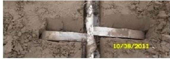
Figure 10a Connection of PVDs to perforated-horizontal pipe
