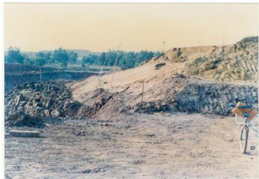
Figure 5 Slope failure of embankment on soft soil
