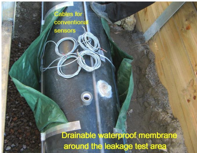
Figure 9 Multi-conduit installation of conventional sensors at centre of test area. Fiber optic conduits 1, 2 and 3 can be seen at left, centre and right respectively. Conduit 4 is located underneath the pipe, approximately below conduit 2
