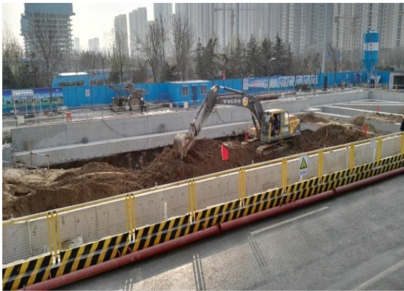
Figure 12 Excavation after First Concrete Support was installed
