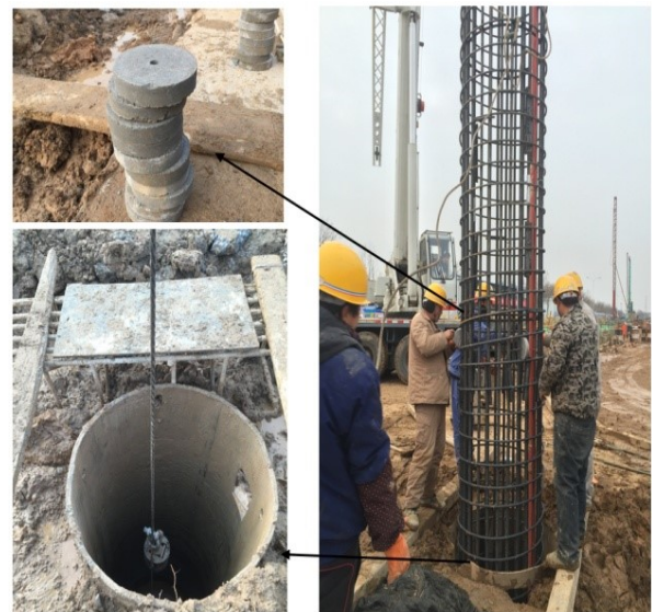
Figure 11 Installation of Steel Reinforced Concrete Pile
