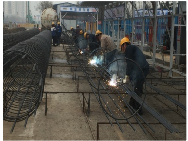
Figure 7 Assembled Steel Cage of Pile
