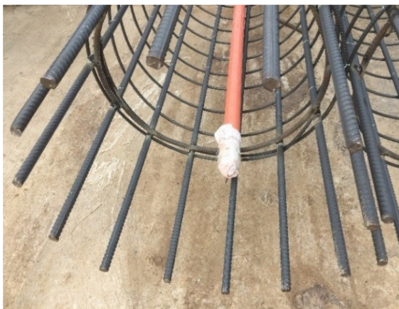
Figure 9 PVC Tube on Steel Cage
