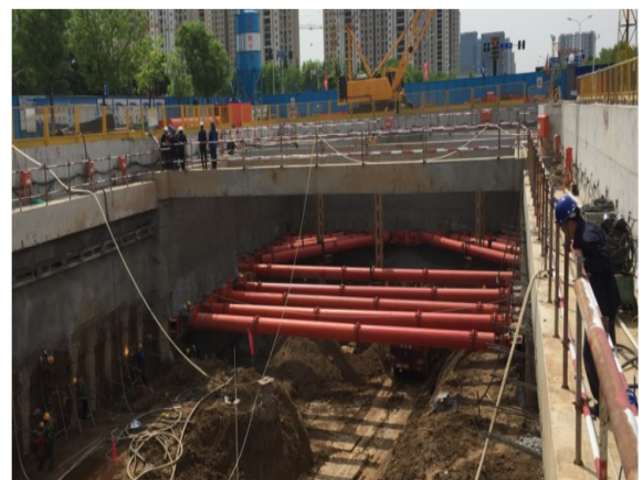
Figure 14 First Steel Support Applications
