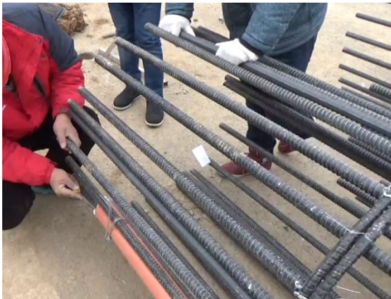
Figure 8 PVC Tube on GFRP Cage
