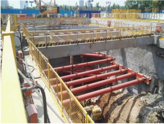
Figure 15 Second Steel Support Applications
