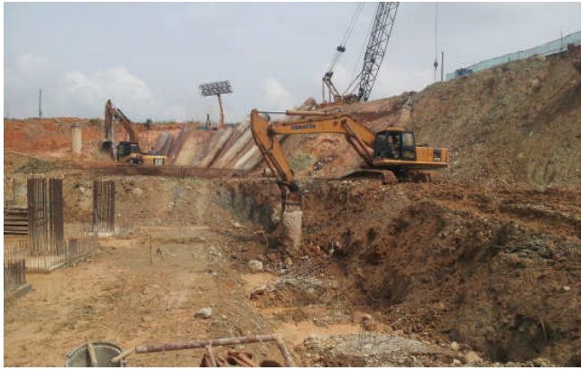
Figure 11 Cut Slope Near Piling Works
