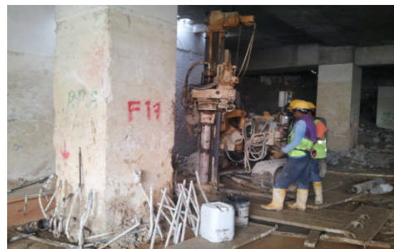
Figure 10 Micropile Rig Working Under Limiting Head Room
