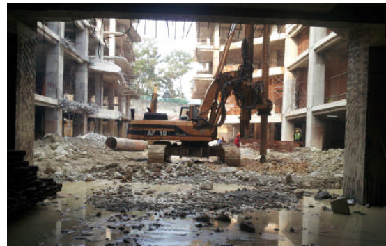
Figure 8 On going Bored Pile Works on Site
