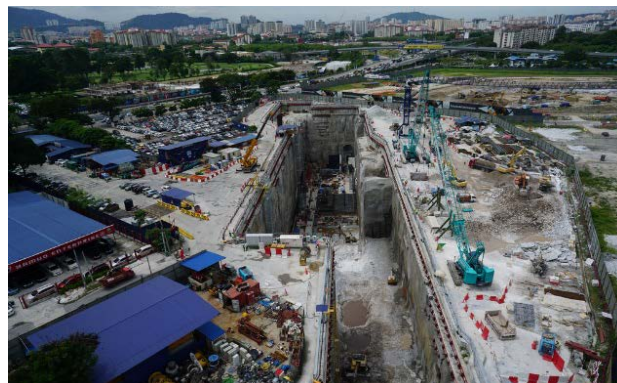
TRX Station with 45m excavation
