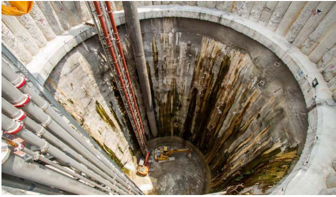
17m diameter Launching shaft
