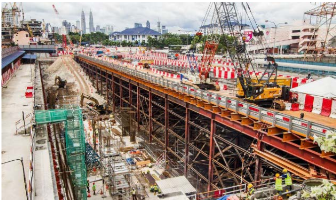
Traffic decking at Maluri Station
