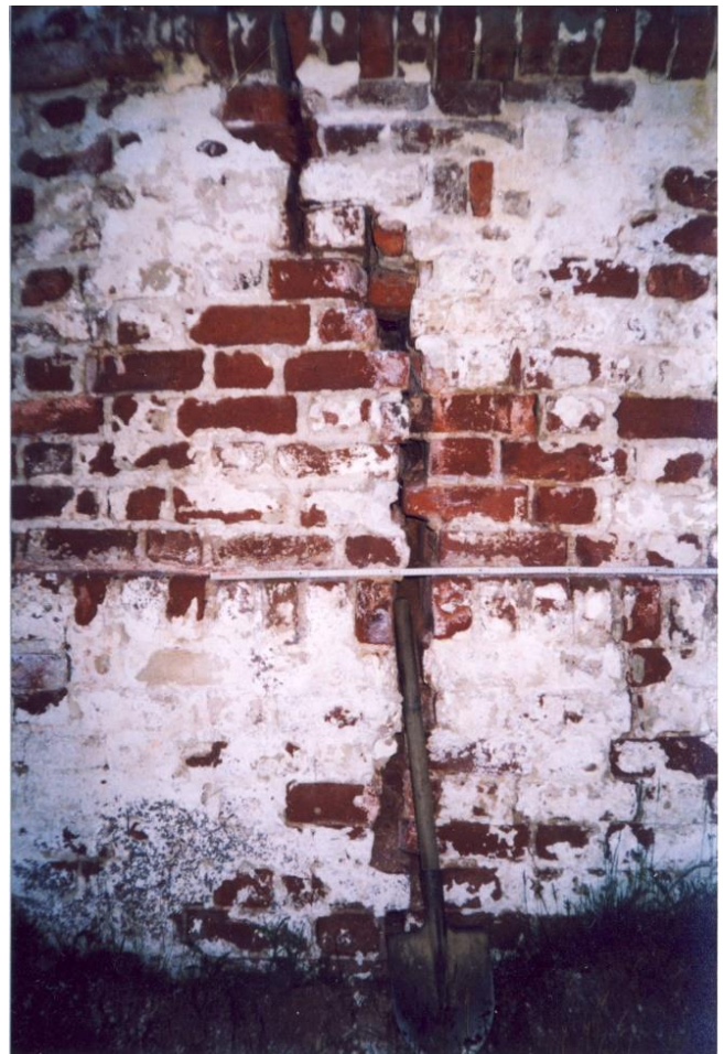
Figure 4 Vertical fracture in the chancel wall, 2000
