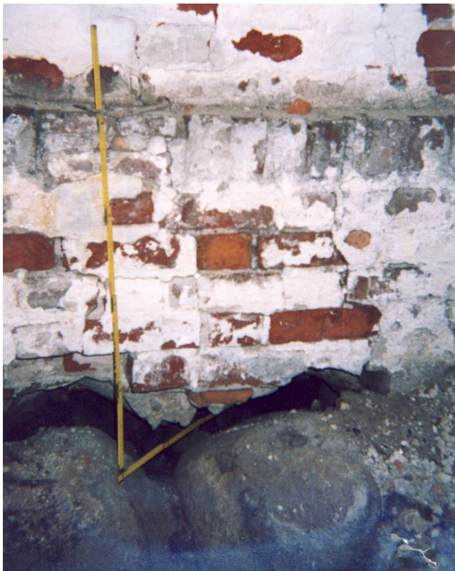
Figure 5 Horizontal fracture of the wall brickwork uplifting from the rubble boulder foundation, 2002
