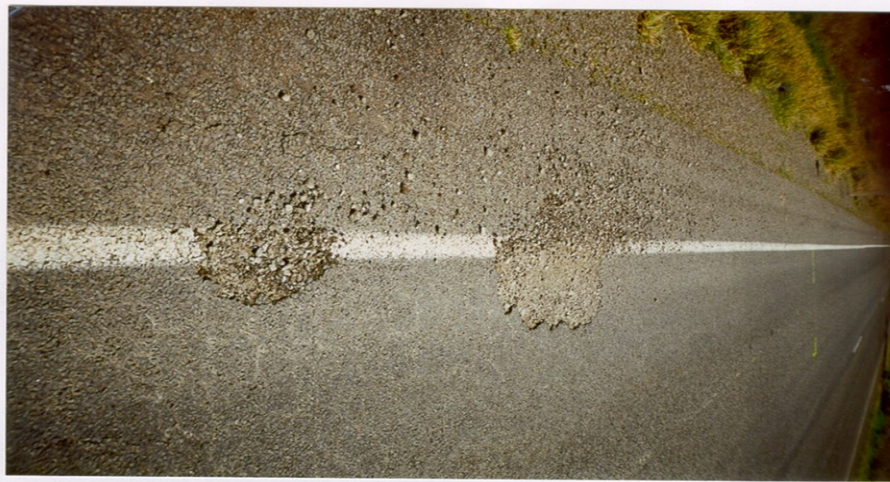
Typical OWP Failures
