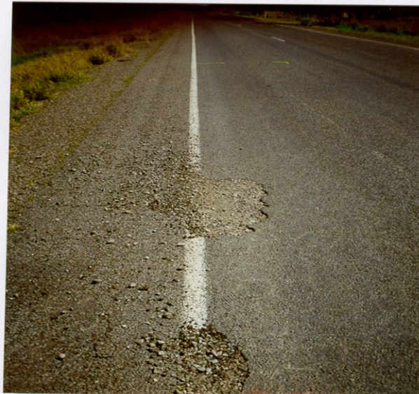
Typical OWP Failures
